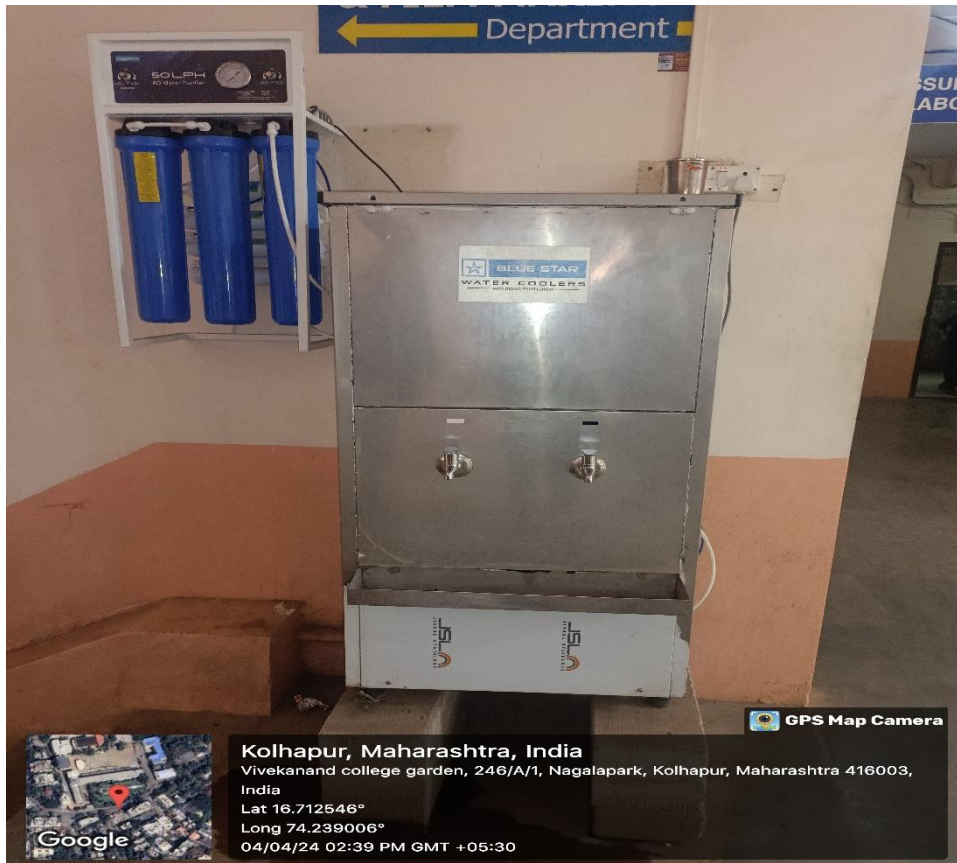
Biotechnology building ground floor filter no.1
