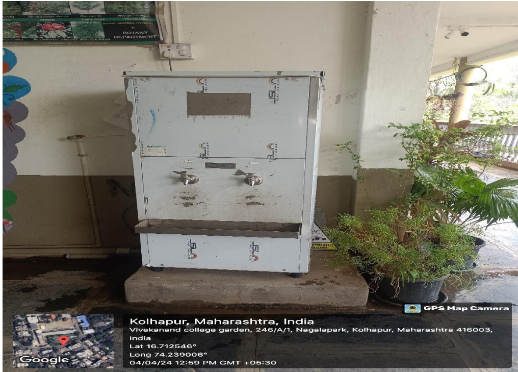
Main building 2nd floor
