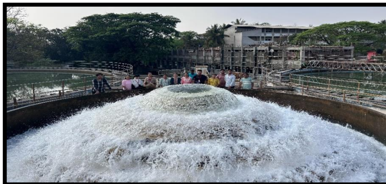
Aeration Tank (Circular type Cascade Aerator) Photos: Field Visit to Sewage treatment plant
